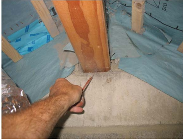
Figure 1. Air leakage detected in the construction phase where improvement is still possible
