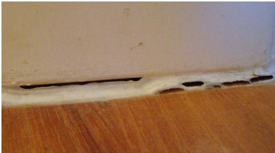
Figure 2. Example of inappropriate choice and placement of a sealing kit resulting in a non-durable airtightness performance
