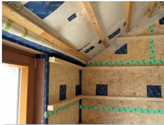
Figure 4. Example of construction where the airtightness layer consists of OSB board
