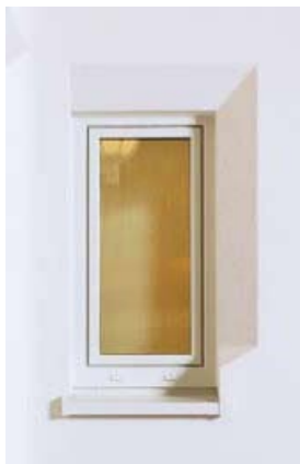
Photo of a Lichtkeil (light wedge) within an externally insulated wall [Copyright KnaufGips KG].
