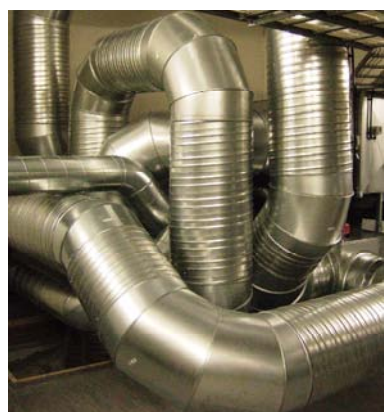
Fig. 2 Circular ducts in a compact Norwegian plant room [foto: SINTEF]
