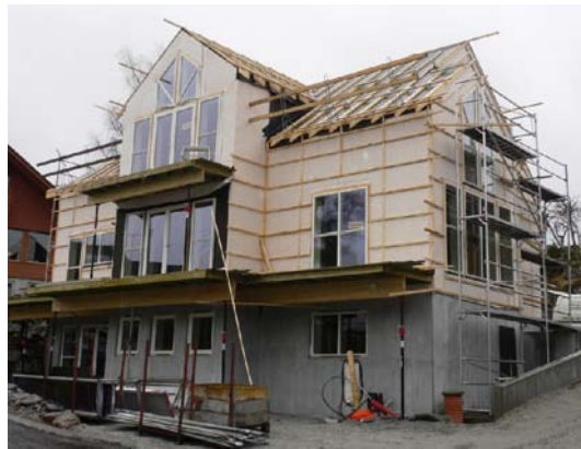
Figure 4 : Building with ambitious details, with a n50-value less than 0.1 /h in early wind-tight stage.
