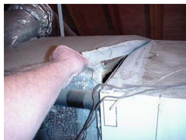
Fig. 1 System with failed tape, and omitted fasteners, in USA [© Weldin Engineering]
