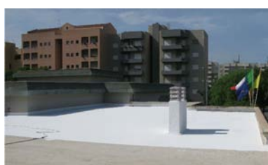
Cool roof coating in a public building in Trapani, Italy.
