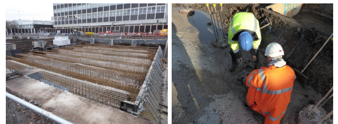
Top: Impression of Energy House 2.0; Bottom: Energy House 2.0 Construction
