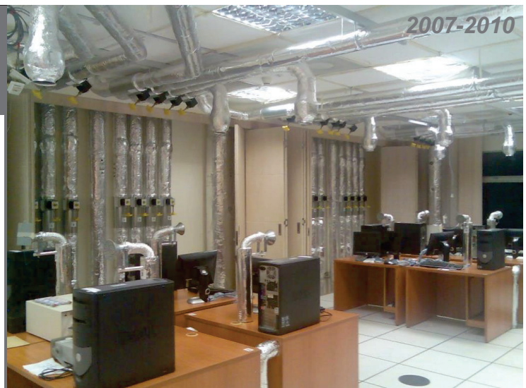
Ceiling-mounted PV system in conjunction with ceiling supply mixing ventilation system
