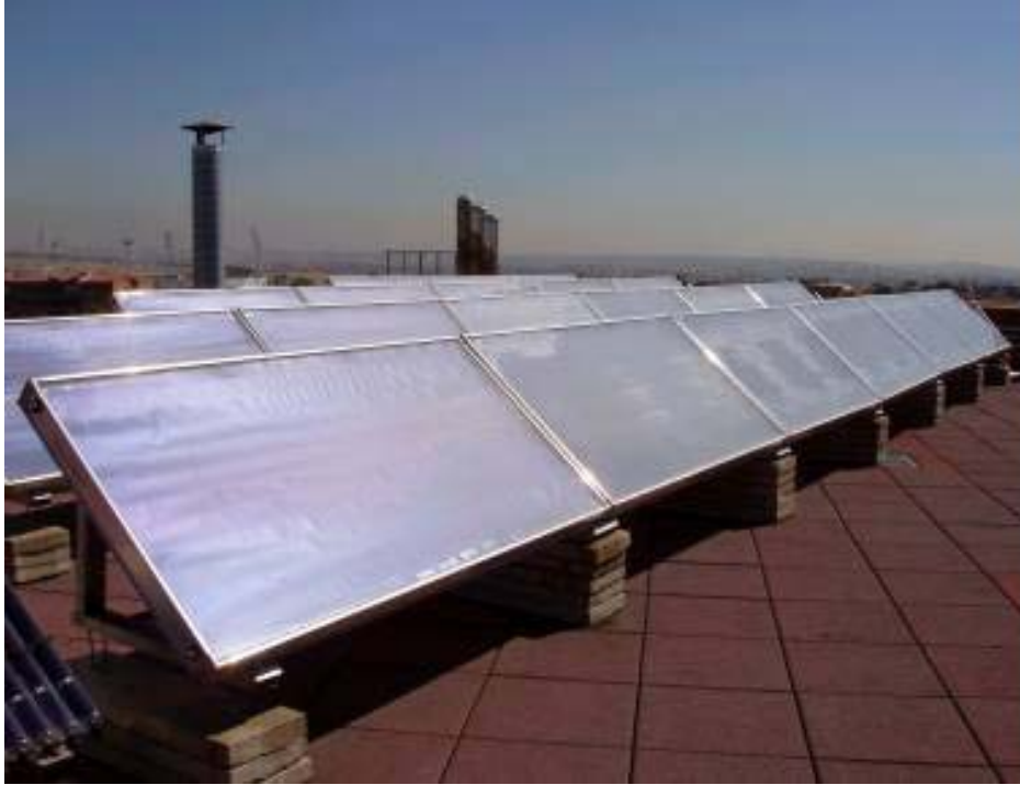
Fig. 2. View of the flat-plate solar collector array installed in UC3M Leganés Campus.
