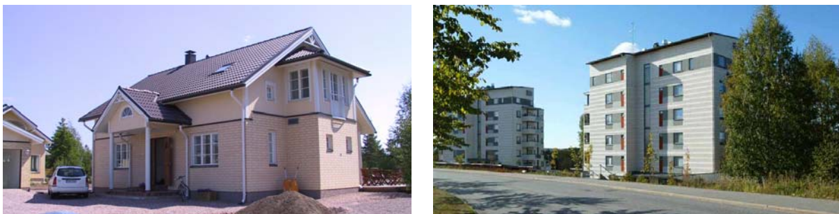
Figure 1 Studied detached house (left) and apartment building (right)
