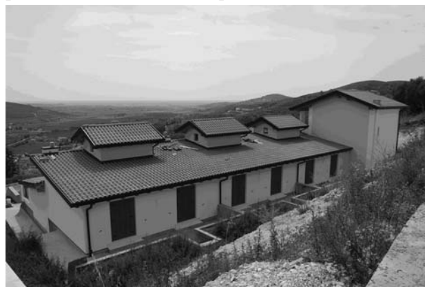
Fig 2. The north façade protected by the hill and with the wind tower for the natural ventilation strategies.
