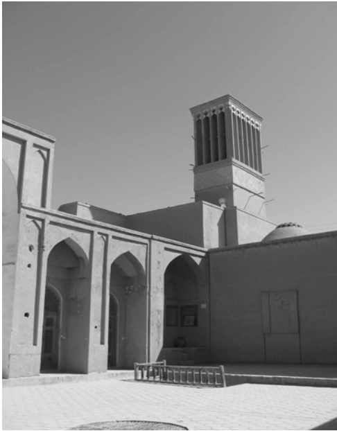
Figure5: Wind catcher in Iranian architecture.
