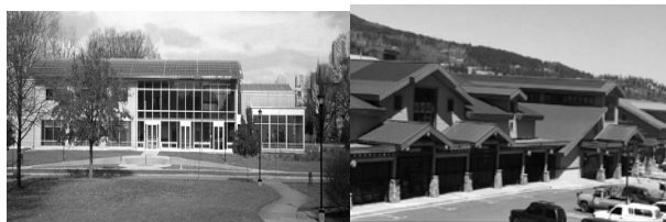
Figure 3: Oberlin College Lewis Center for Environmental Studies (left), Bighorn Home Improvement Center (right) (Hayter et al., 2002).
