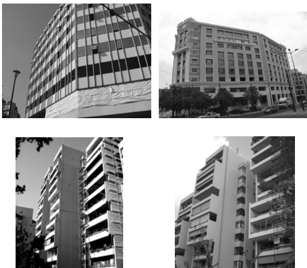
Figure 4a, b, c, d: Project A& B before/after renovation.
