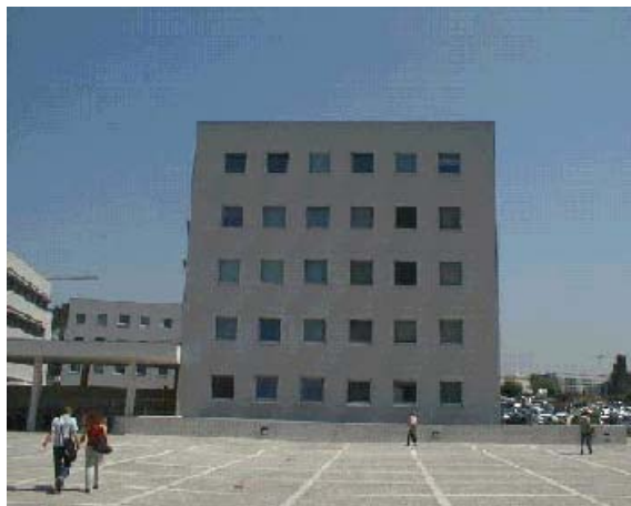
Figure 16a. Office building (external view).
