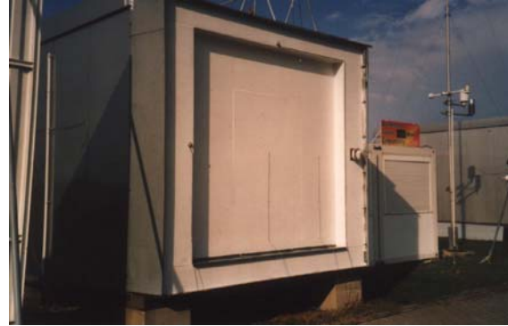
Figure 2. Opaque wall installed in PASLINK test cell at BTU Cottbus, Germany.
